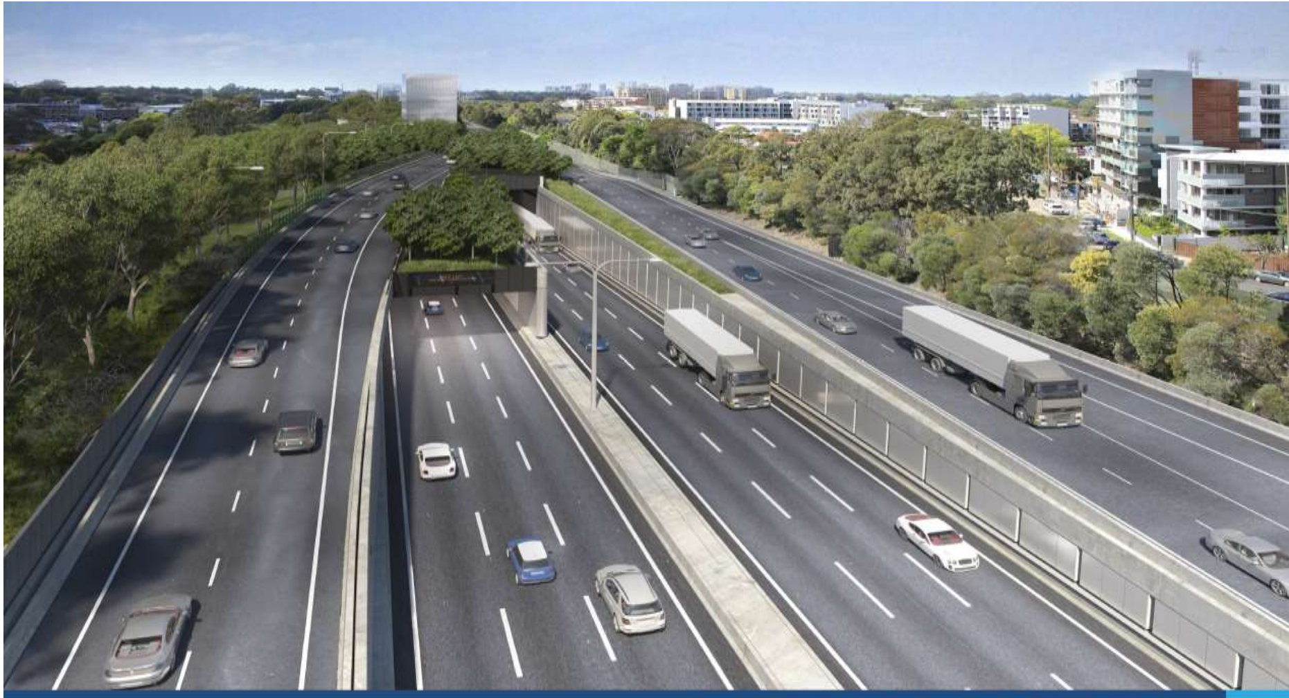
Homeshush Bay Drive Interchange - Aerial view of proposed tunnel portals (Artists impression only)
